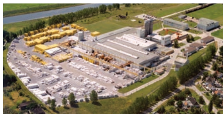
Calbe Factory, Germany
